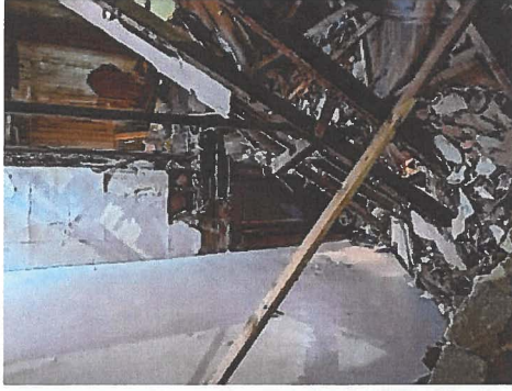
EXISTING INTERIOR STAIR TO BASEMENT
