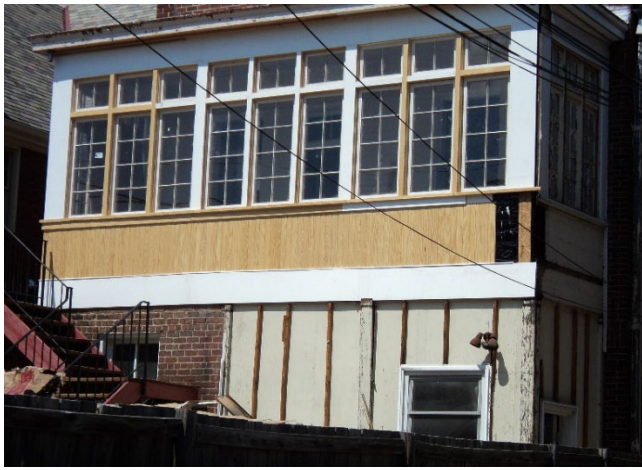
Figure 2. Replacement windows being installed on the sunroom, 2015.
