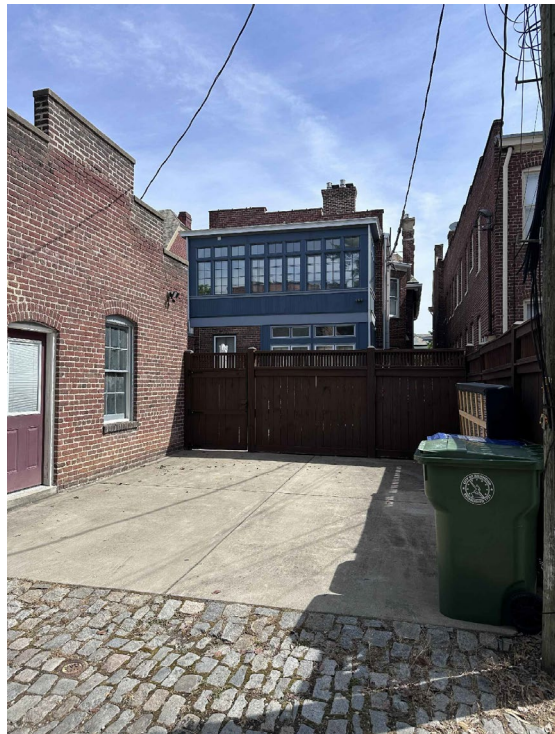
Figure 5. Existing conditions at rear of monument Avenue.
