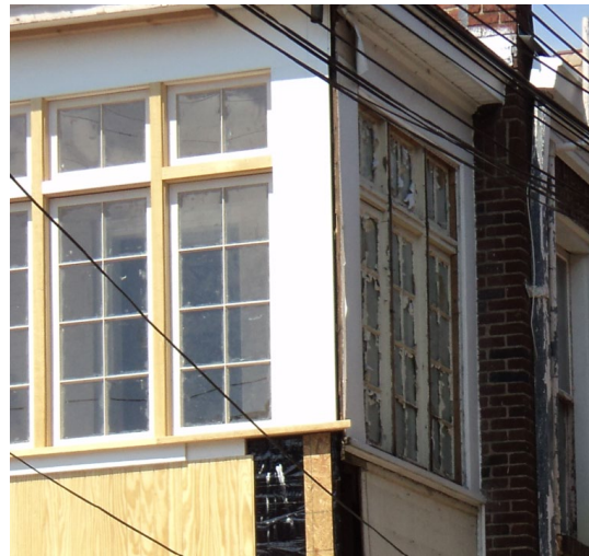
Figure 3. View of sunroom in 2015 rehabilitation. East elevation windows are visible as being repaired and salvaged, while south elevation windows are new.
