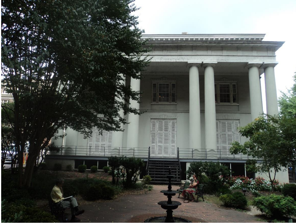
Figure 10: Rear Elevation of White House of the Confederacy viewed across the garden
