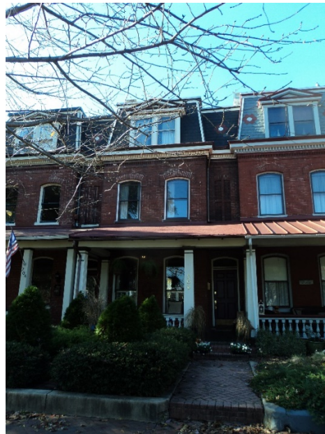
Figure 2. Facade of main building.
