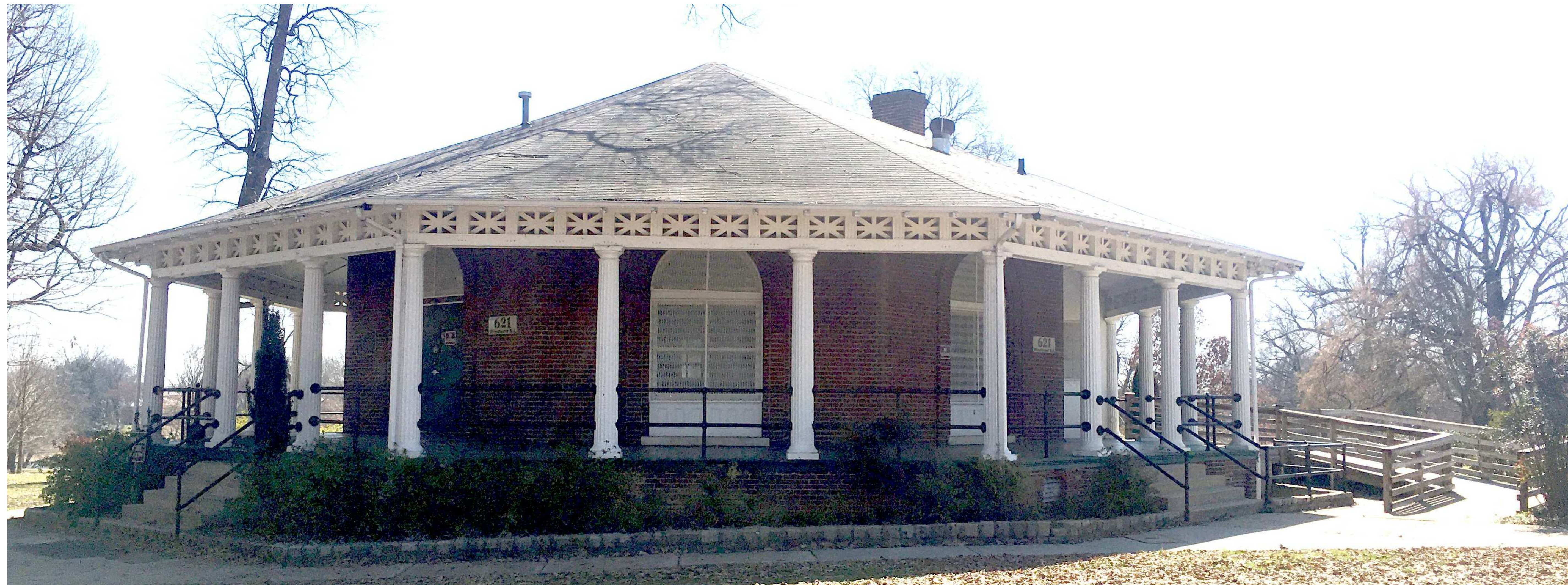
EXISTING NORTHWEST FACADE
