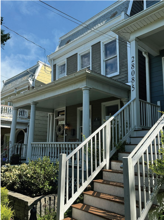
Figure 1. Front Façade with narrow siding.
