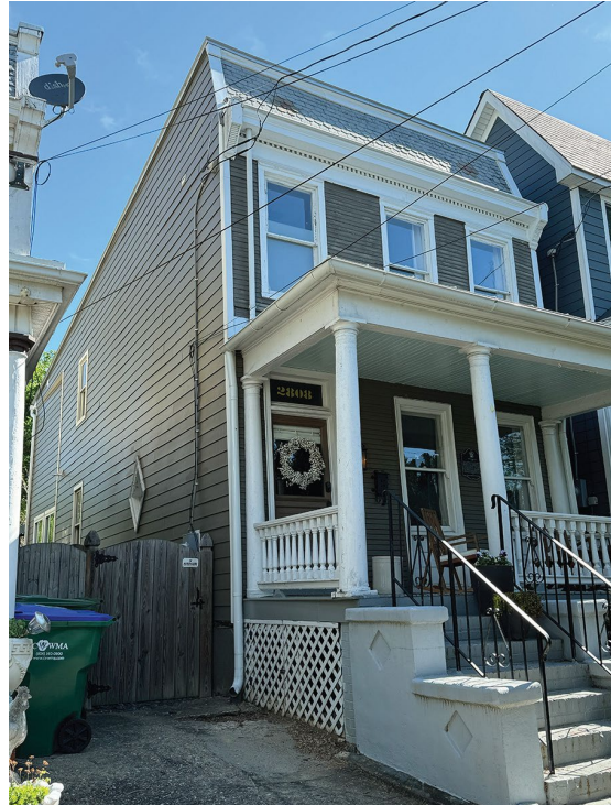
Figure 2. Side façade with replacement siding.
