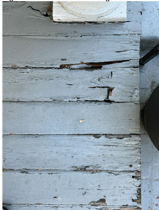
Figure 6. Deteriorated decking boards.
