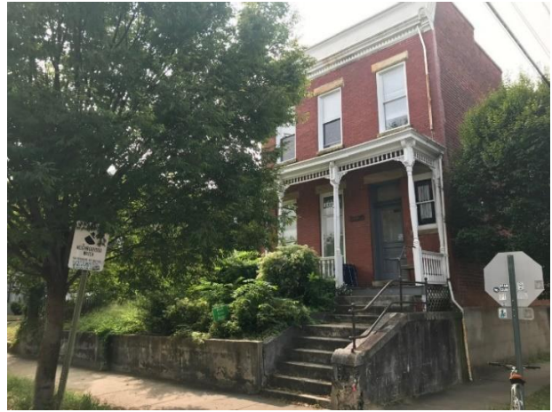
Figure 2. 3135 W. Franklin Street, existing building on the lot.
