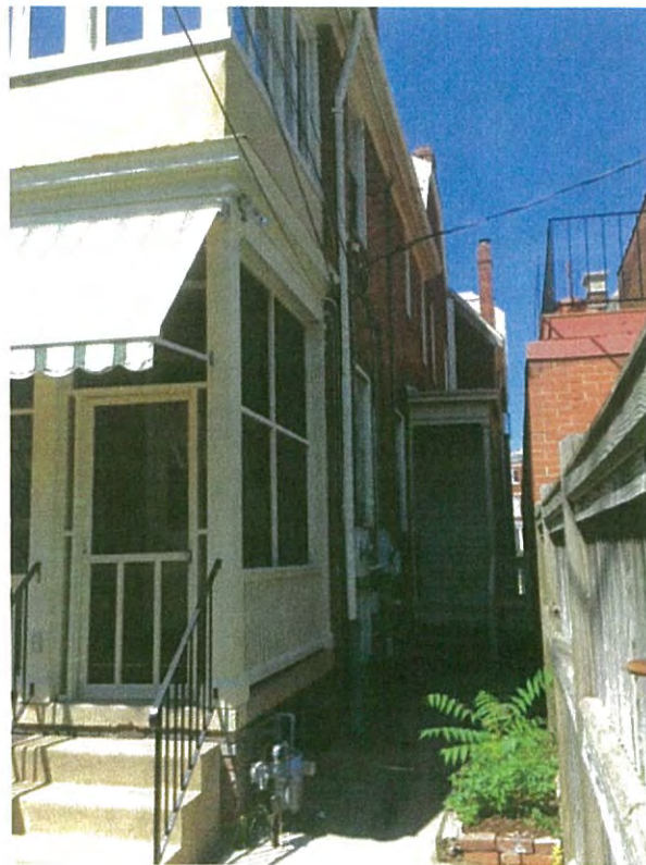
Back porch and side of back porch from patio
