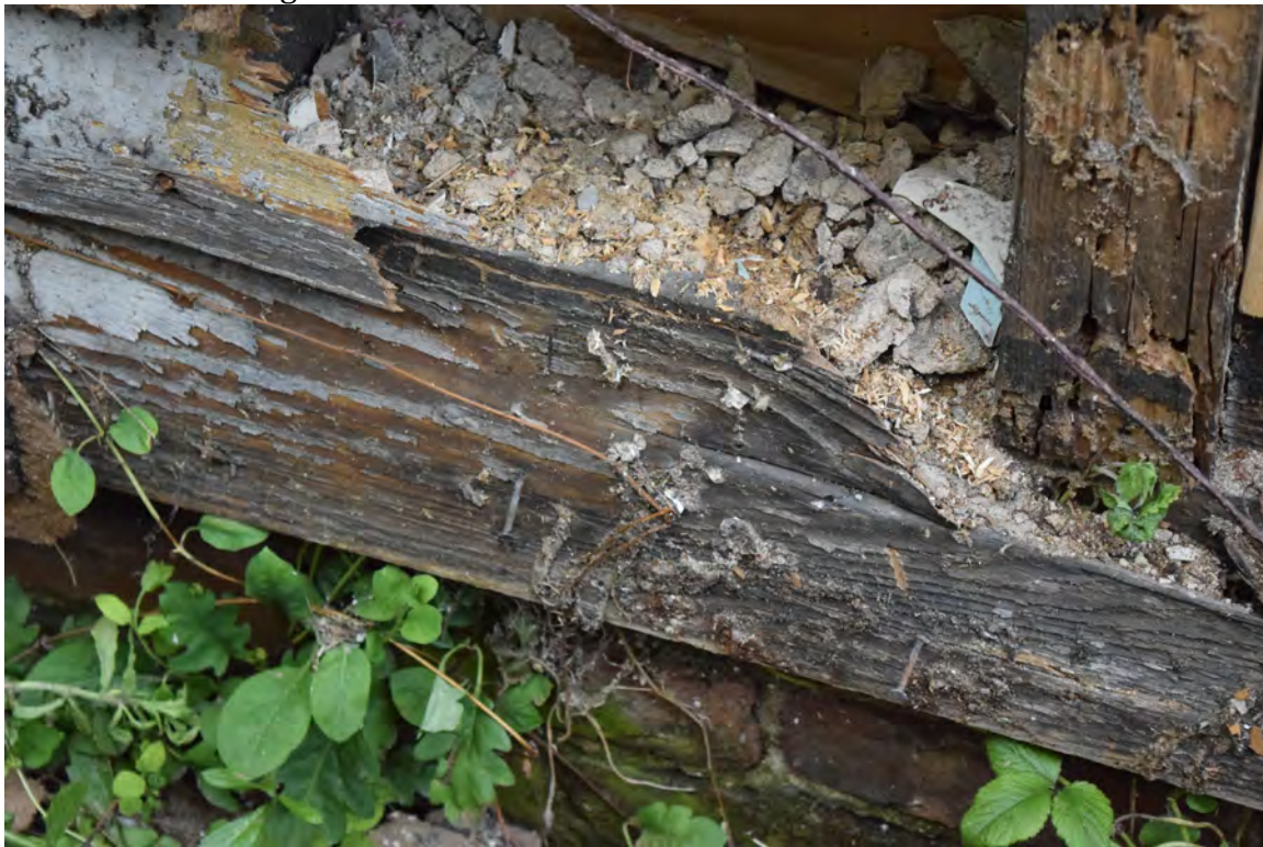
Rotten Wood Siding Photos:
