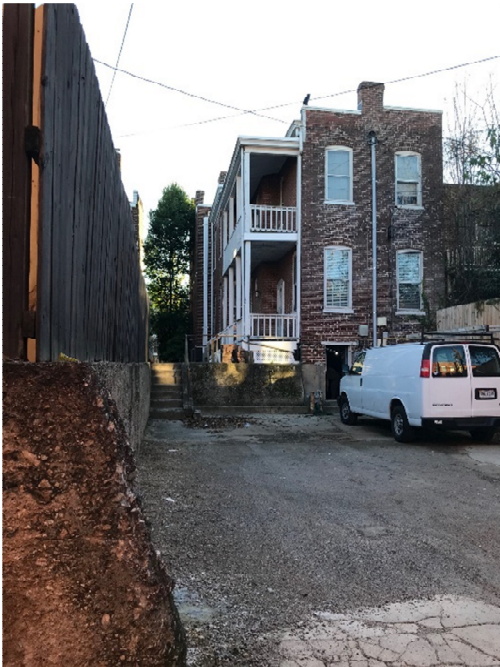
Figure 3. 2204 West Grace Street, rear walk and stairs.
