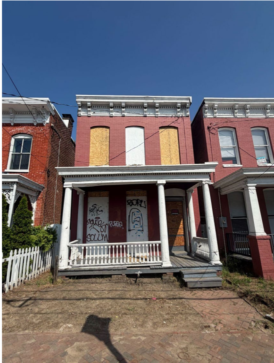
Figure 1. Existing conditions. Facade of 606 North 1st Street.
