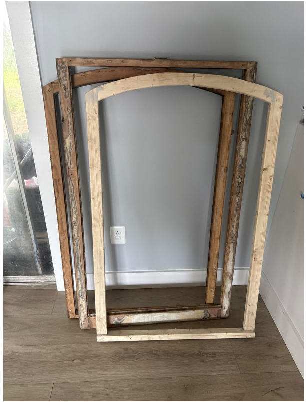
Figure 6. Arched windows being reconstructed to be reinstalled on the facade.
