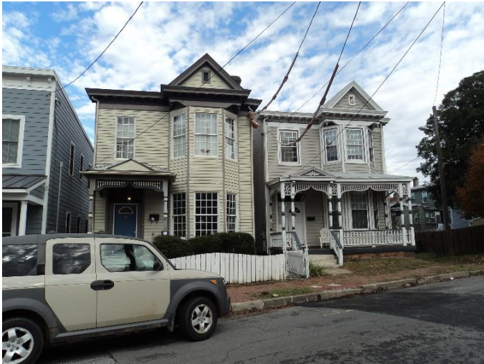
Figure 7. North side of 2000 block Cedar Street, looking north
