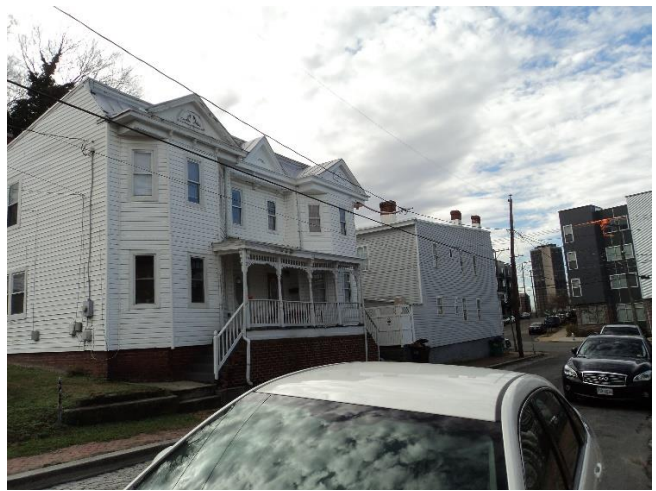
Figure 4. South side of 2000 block Cedar Street, looking southwest
