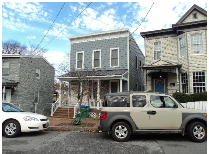
Figure 6. New construction, 2008 Cedar Street
