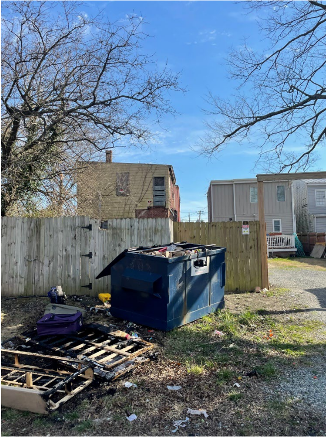
Figure 7. Rear elevation from public right-of-way
