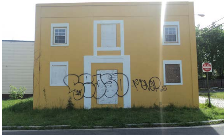
Existing Condition of the Façade of 815 North 22 nd Street
