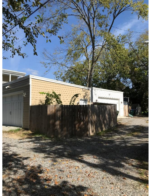
Figure 4. New construction outbuildings on the subject block.
