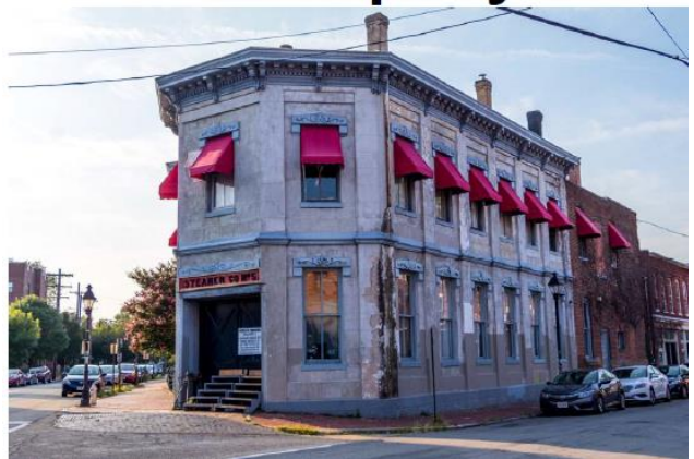
Figure 4. 200 West Marshall Street, Brook Road elevation.
