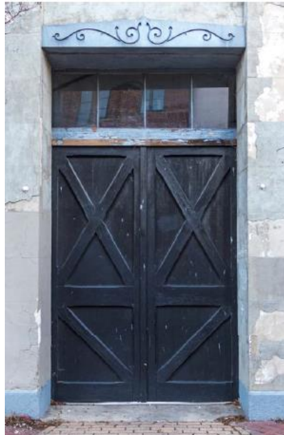
Figure 6. Door 2, second floor entry door.
