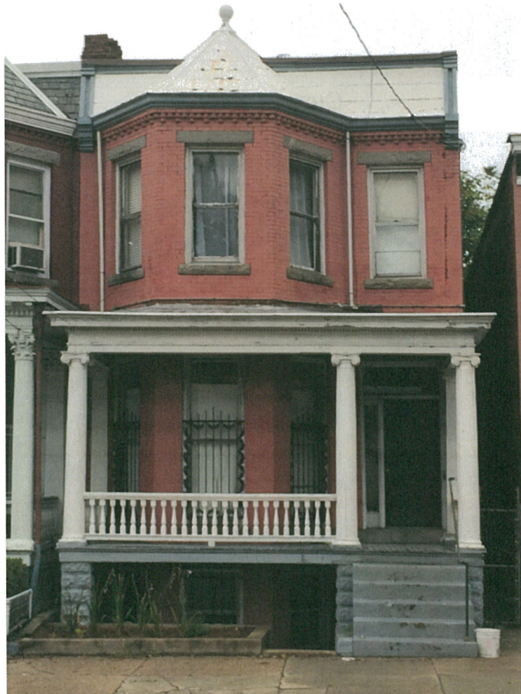
Current photograph from street
