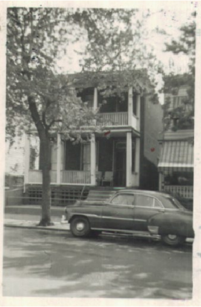
. Figure 6. Original dwelling on-site. Demolished
