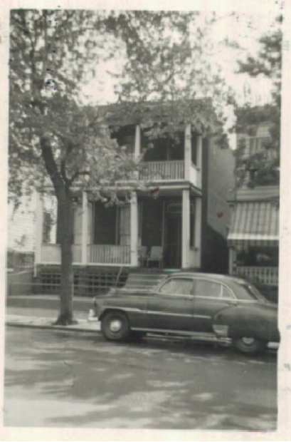
. Figure 6. Original dwelling on-site. Demolished
