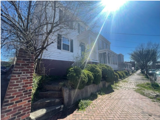
Figure 1. Subject block looking south.
