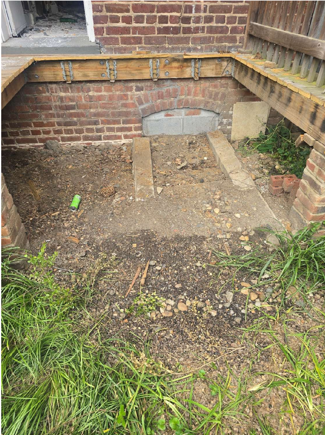
Infilled masonry basement door opening and side walls of steps
