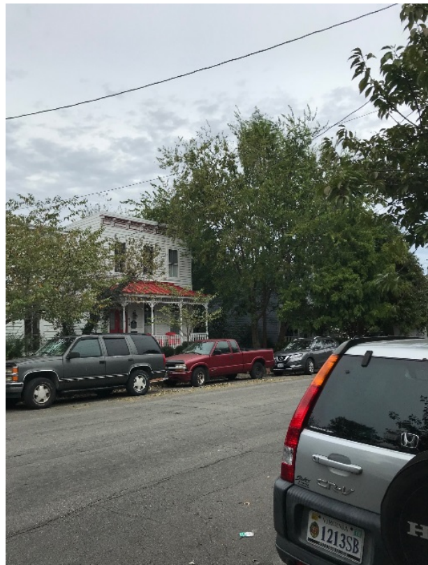
Photograph 2. 418 North 23rd Street, current conditions.
