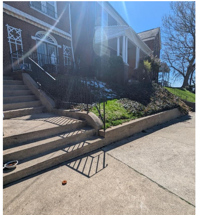
Figure 4: Concrete curb and steps on adjacent lots, that appear to be original
