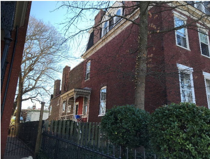
Figure 3. View of north elevation from North 29th Street.
