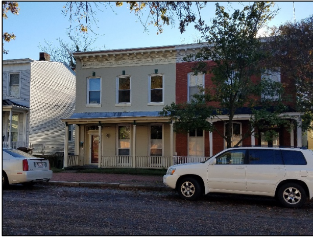
Figure 3. 305 N. 30th Street.
