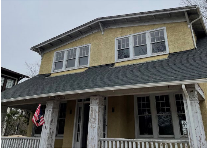
Figure 3. New asphalt shingles, 3833 Hermitage Road (After)
