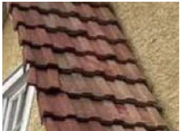
Figure 7. Original Concrete Tile with French profile
