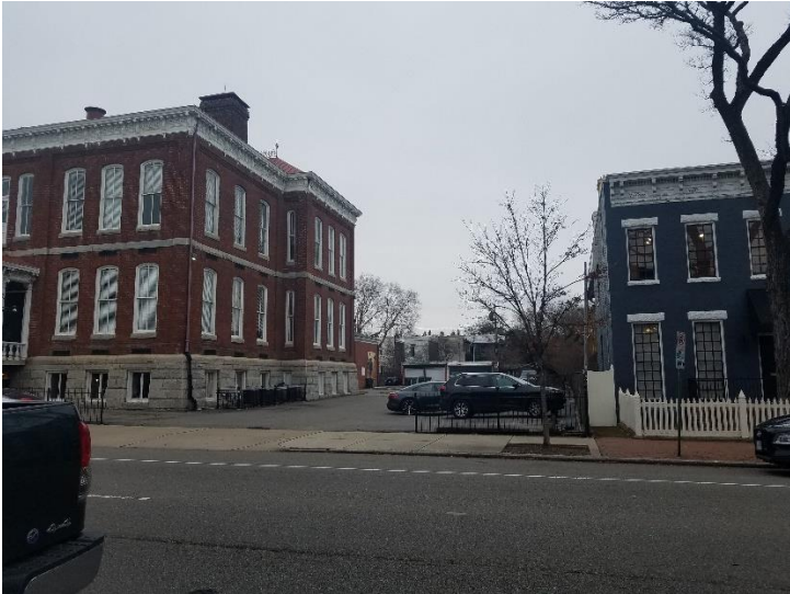
Figure 1. 1518 West Main Street
