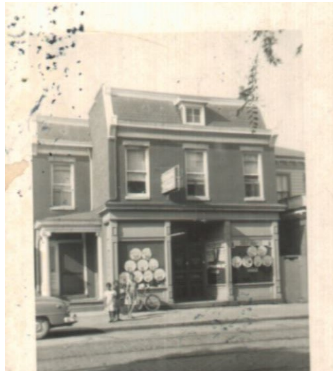
Historic Front Elevation of 3103-3105 East Marshall St.
