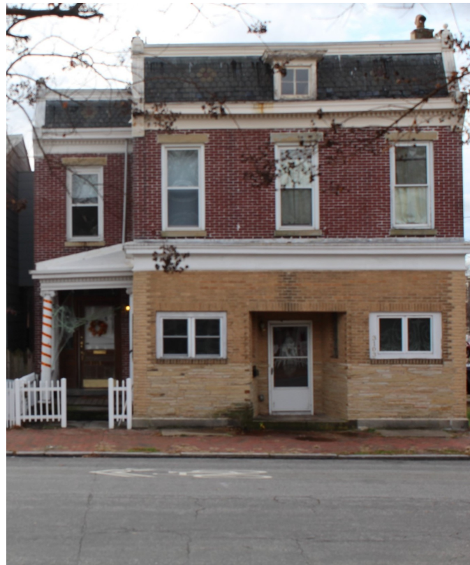
Existing Front Elevation of 3103-3105 East Marshall St.
