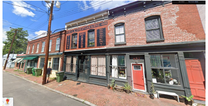
Figure 3. Primary entrances along Brook Road that feature a wooden, stone, or concrete step.
