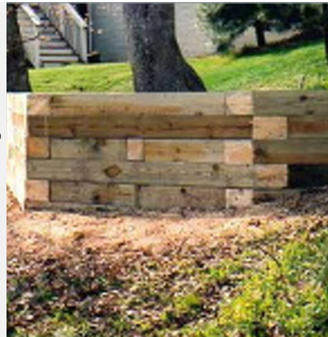
Timber Retaining Wall
