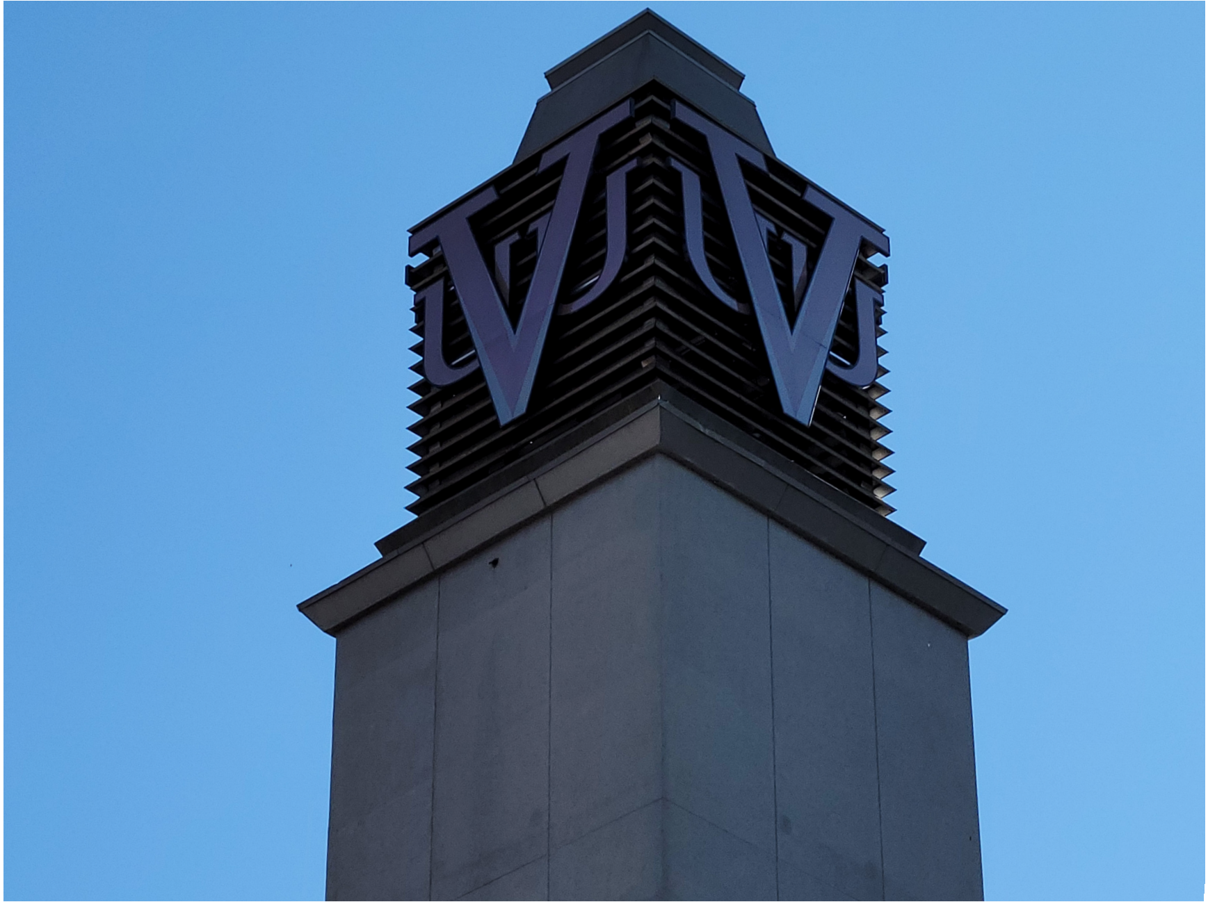
North and West Exterior Detail
