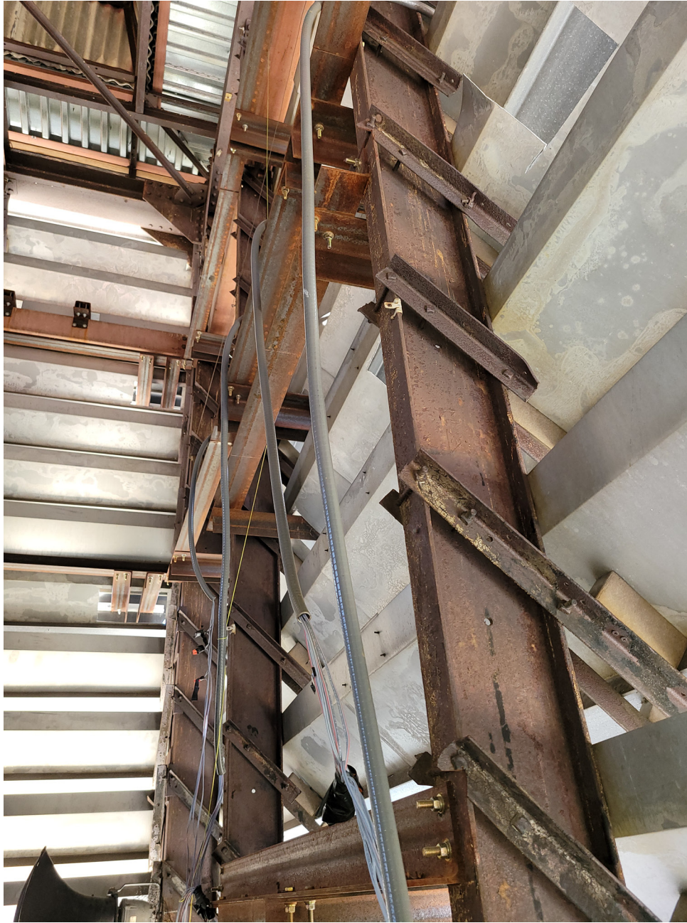
Existing and New Connection Details
