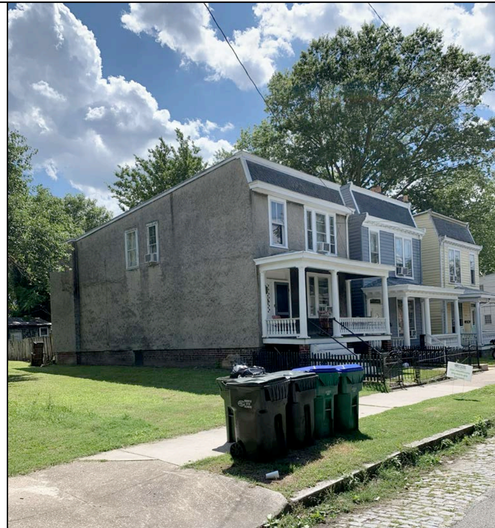
VIEW OF SITE & NEIGHBORING HOUSES
