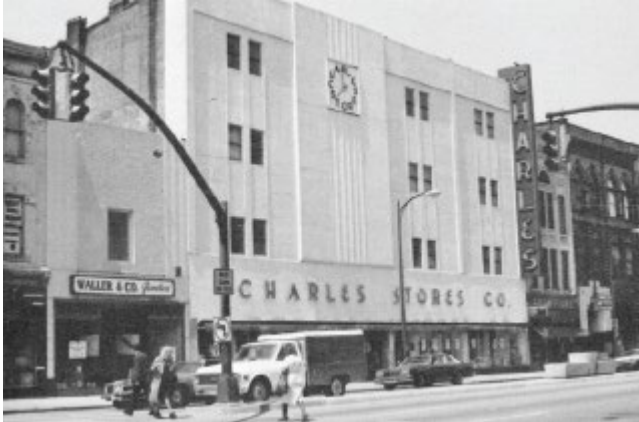
Figure 2. Original building after front façade alterations. Demolished 1989
