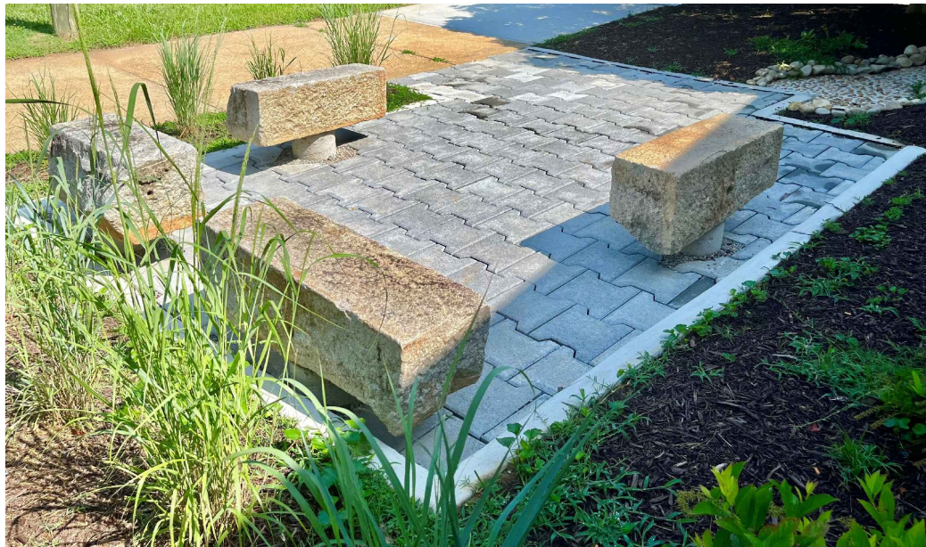
Reclaimed granite benches and Powerblock pervious pavers
