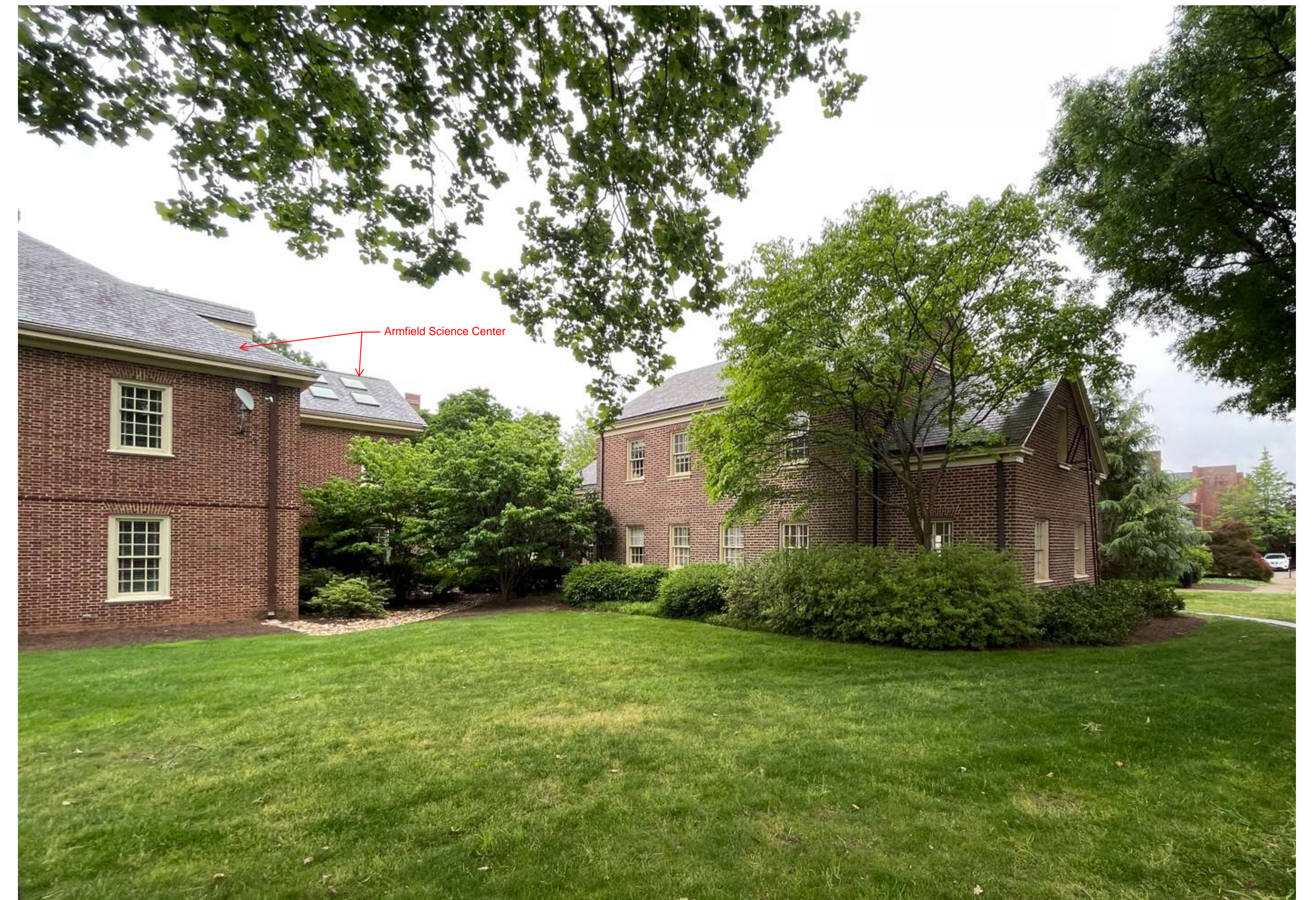
Existing North Facade and Courtyard - location of proposed addition
