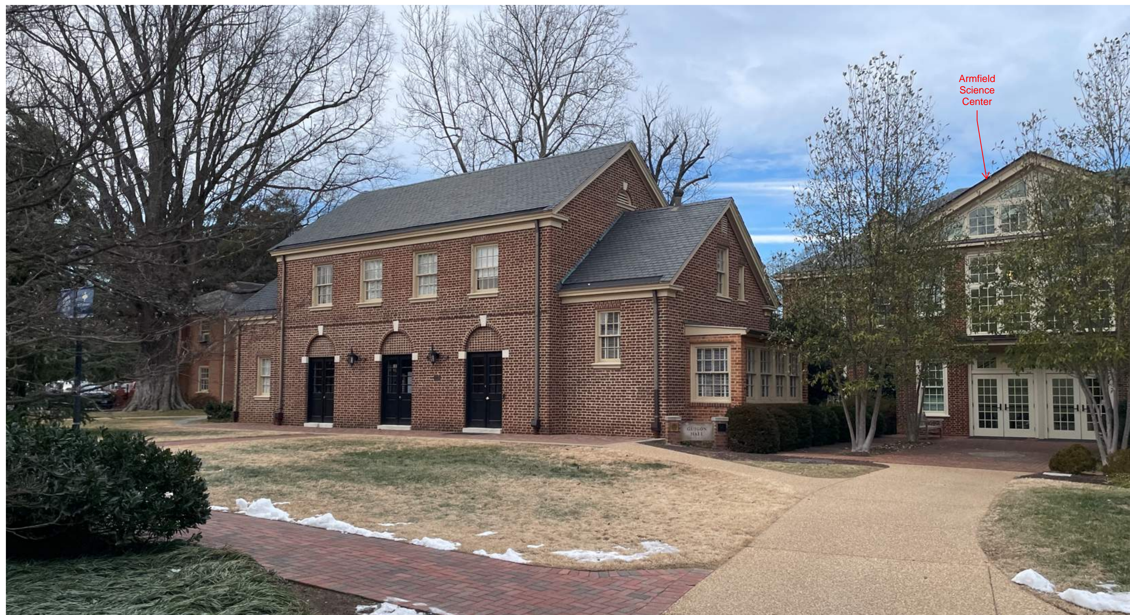
Existing Southeast Corner - showing existing adjacency to Armfield Science Center entrance
