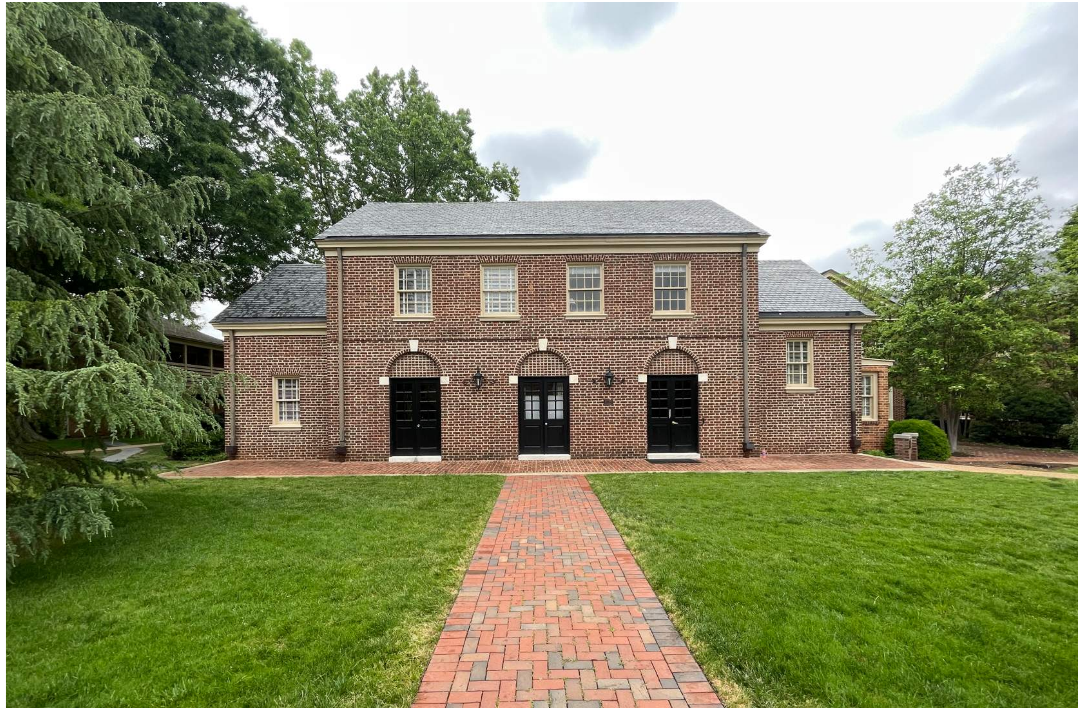
Existing South Facade - campus-facing, historic entryway - to be preserved through the renovation
