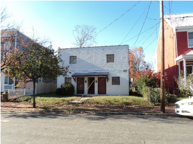
Figure 1. Existing front elevation of structure.
