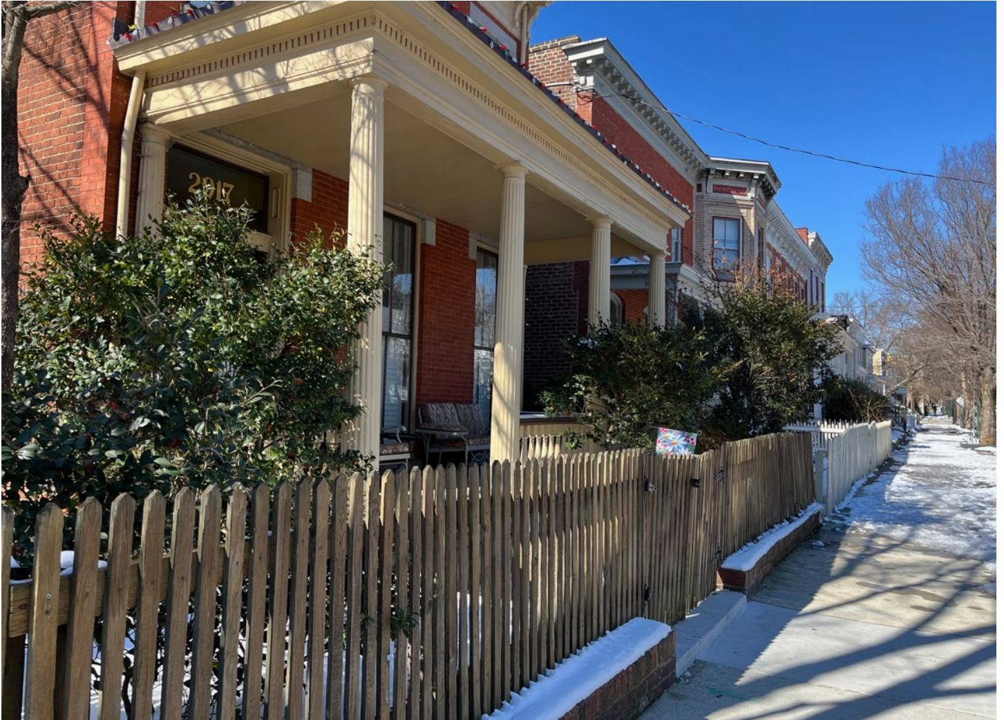
Figure 3. Subject property, looking west down East Broad Street.
