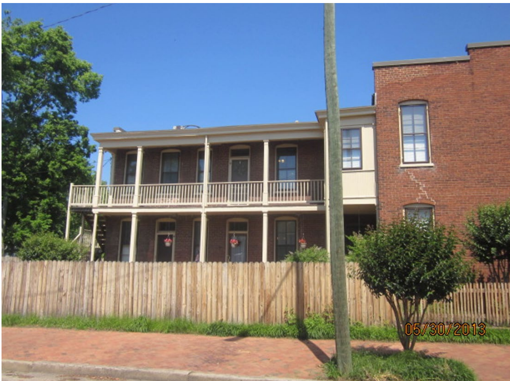
Figure 2. Extant side wooden privacy fence.
