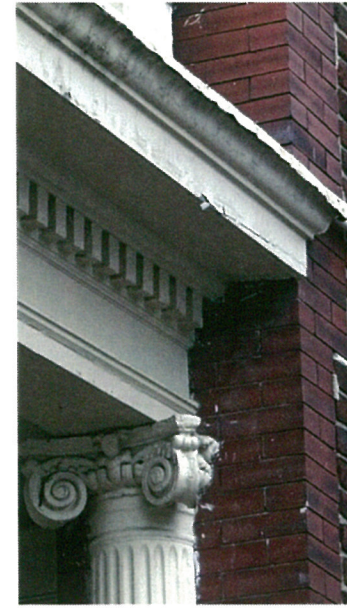
Eave & Railing Shadow 2211 Hanover Avenue
