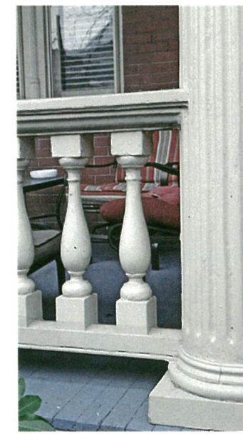
Baluster & Railing 2211 Hanover Avenue
