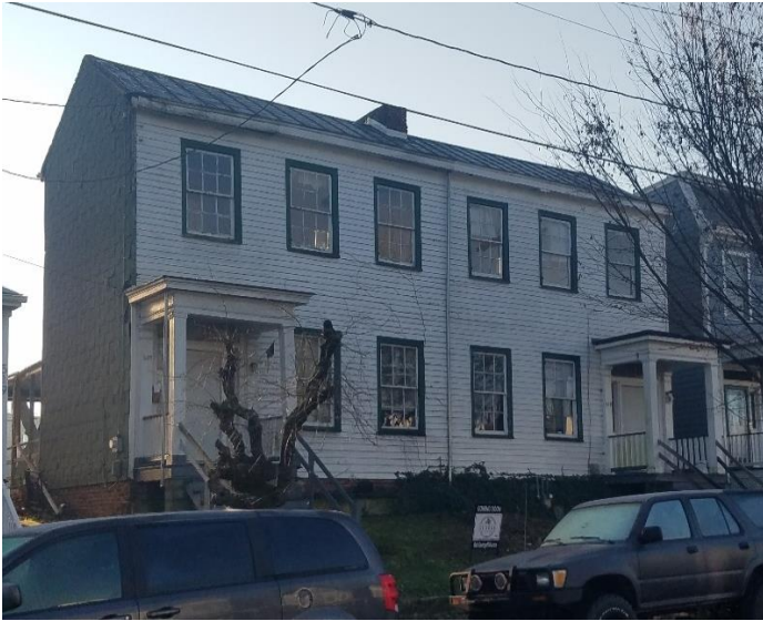
Figure 1. 515-517 North 28th Street, façade
