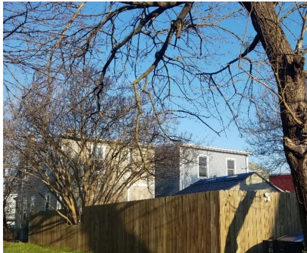
Figure 4. Rear massings on subject alley
