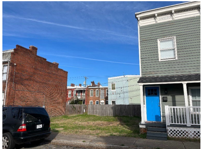
Figure 4. Subject lot at 2316-2318 Burton Street.
