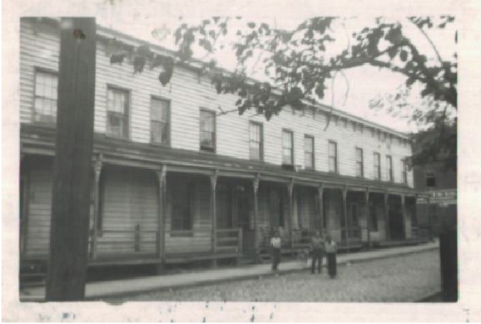
Figure 1. Assessor's Card photo showing the attached dwellings located at 2316-2326 Burton Street. The end units located at 2316-2318 Burton Street, the subject parcel's buildings were demolished sometime in the late 1970's or early 1980's.
