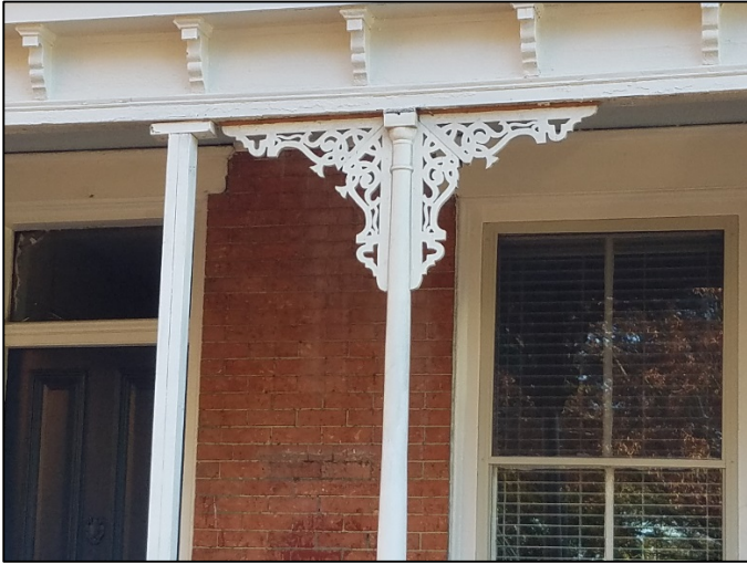
Figure 7. Front porch bracket detail.
