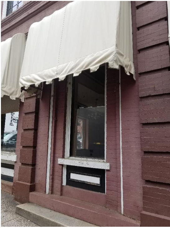
Figure 5. East Cary Street window to become a door.
