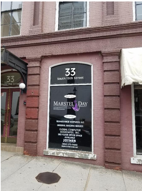
Figure 3. South 13th Street window to be replaced
