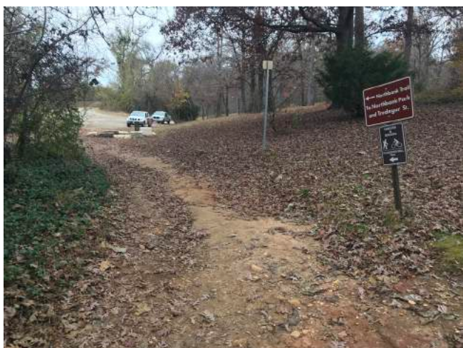
Existing footpath to be removed and the area reseeded. Signs to be relocated.
