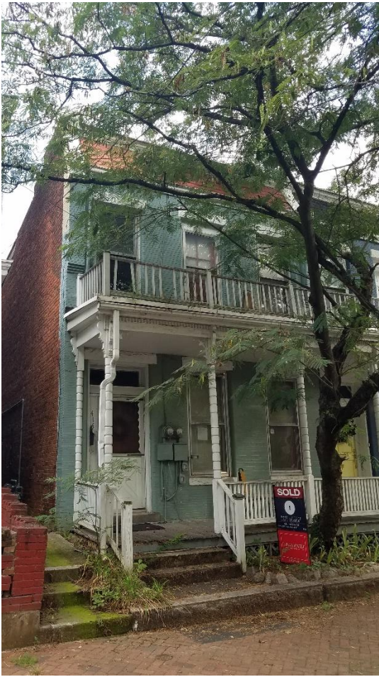
Figure 1. 414 N. 27th Street, façade.
