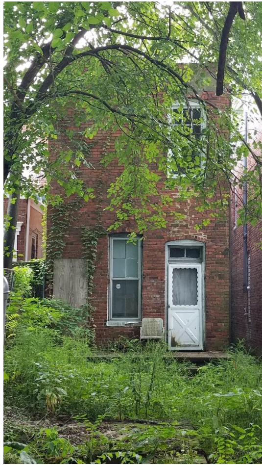
Figure 2. 414 N. 27th Street, rear elevation.
