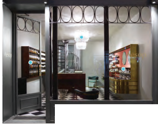
STOREFRONT Black or Dark Bronze Anodized Aluminum Frame w Clear Insulated Glazing
