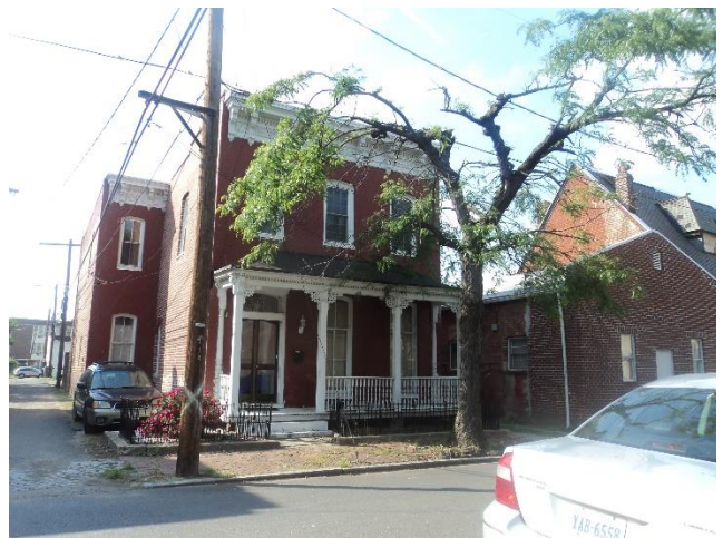
Figure 4. 500 block St. James St, even side
