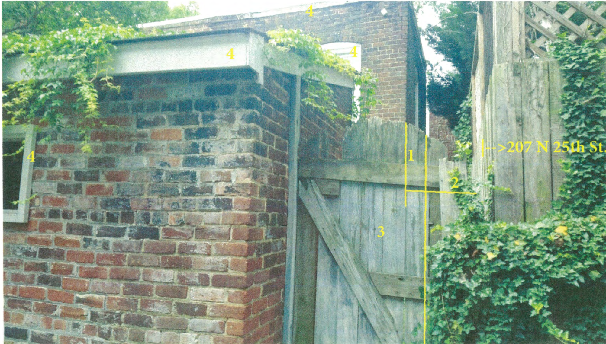
Photo 2: Rear from NW Corner (Alley View)
