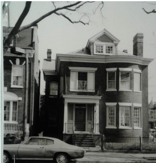
Figure 2. 401 North Allen Avenue, façade ca. 1980
