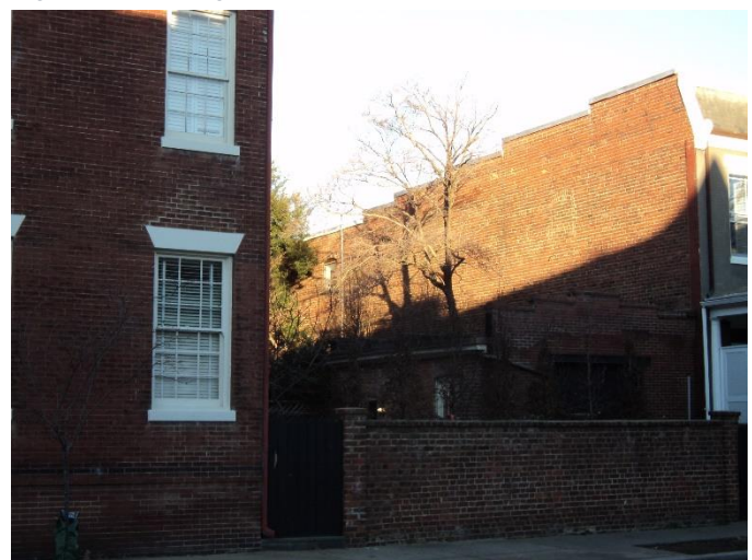
Figure 6. View of garage openings from Park Avenue
