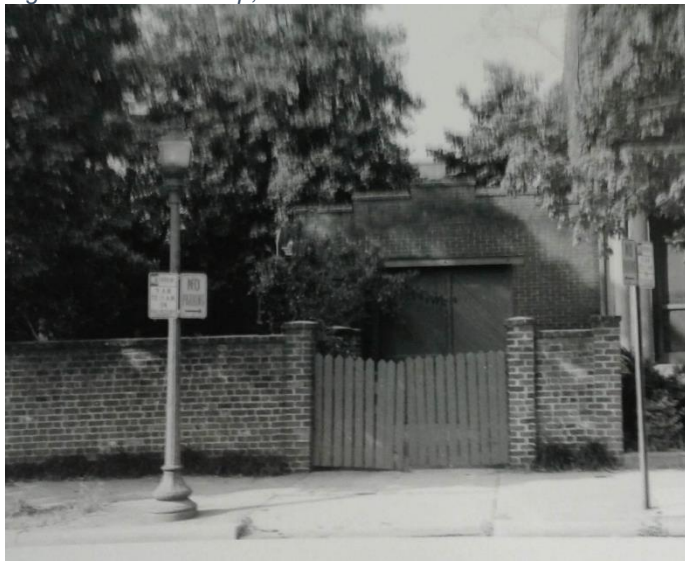
Figure 3. 401 North Allen Avenue, ca. 1980, garage in rear
