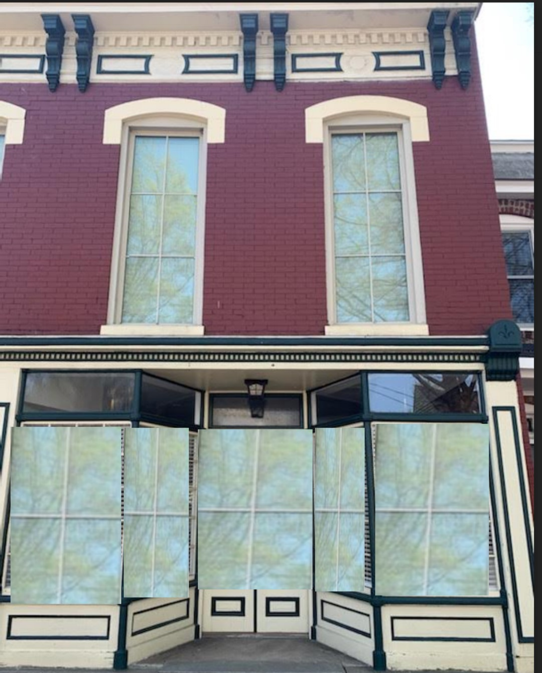
Southern door removal with windows to match second floor
