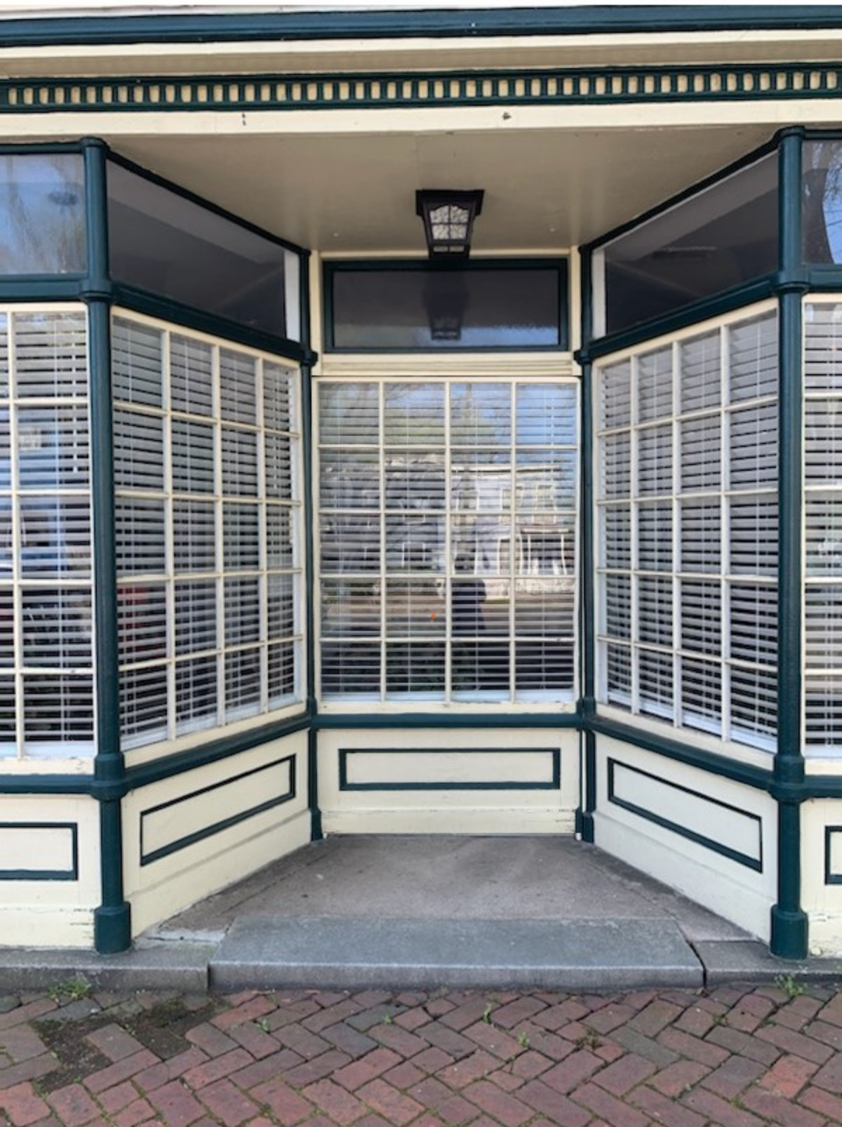
Southern door removal
