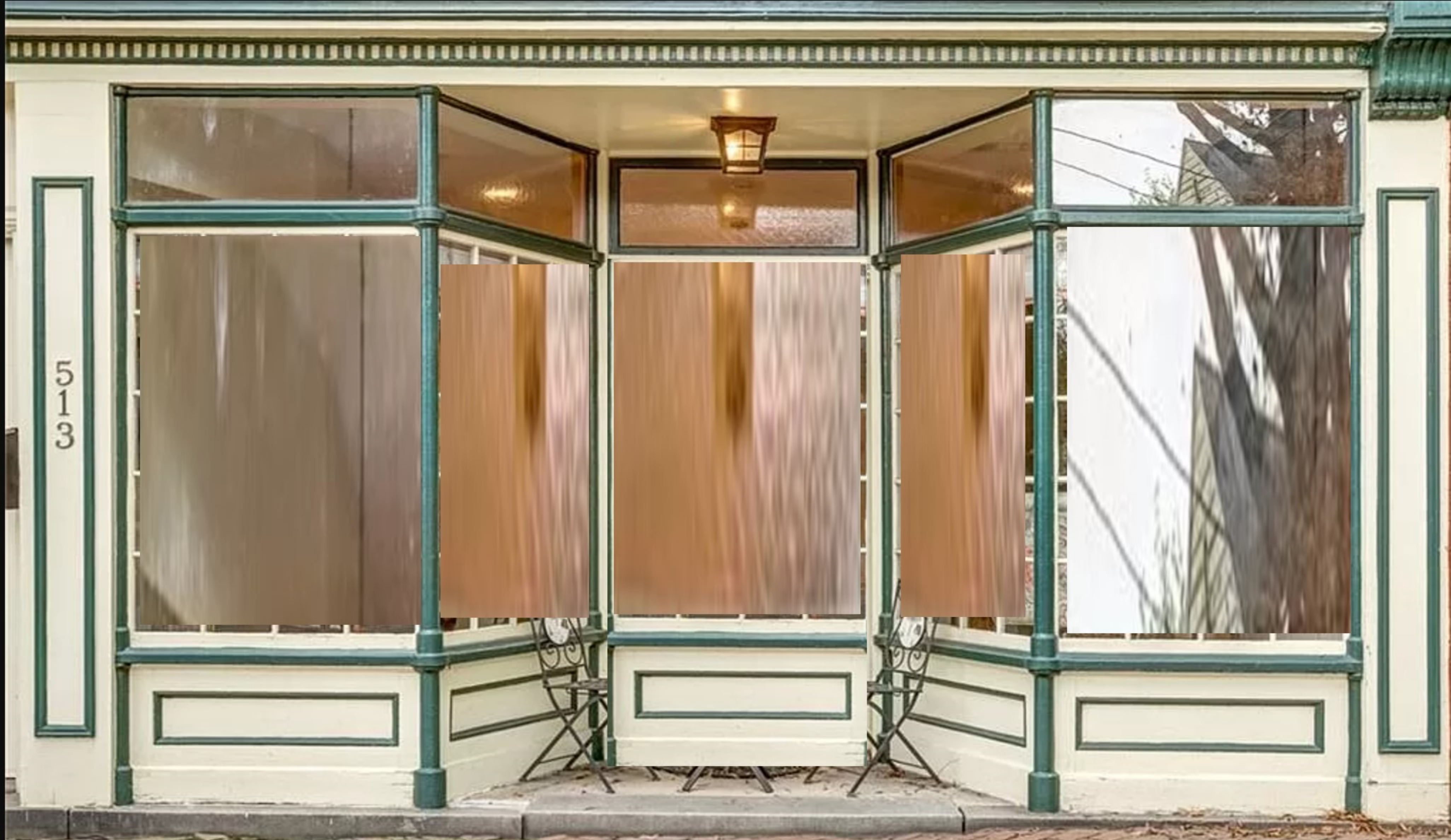
Southern door removal with full picture window
