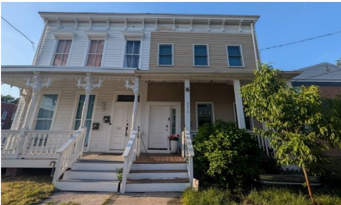
Figure 2: Example of a Cornice treatment
