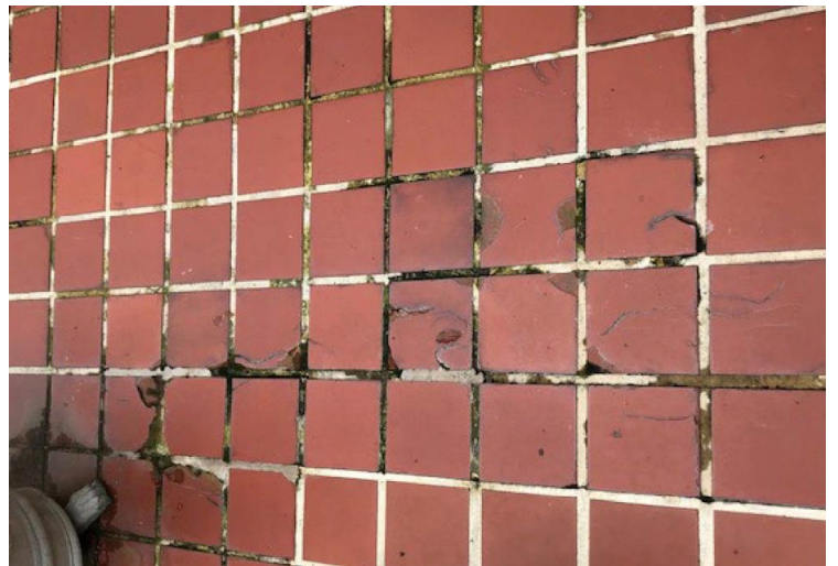
Figure 4. Existing tile on patio
