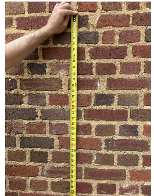
Existing brick & mortar to be matched
